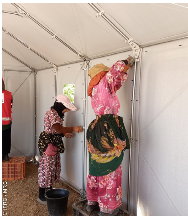
Staff and volunteers received training on TSU installation, and over time could install two or three units daily, compared to one unit per day at the start.
