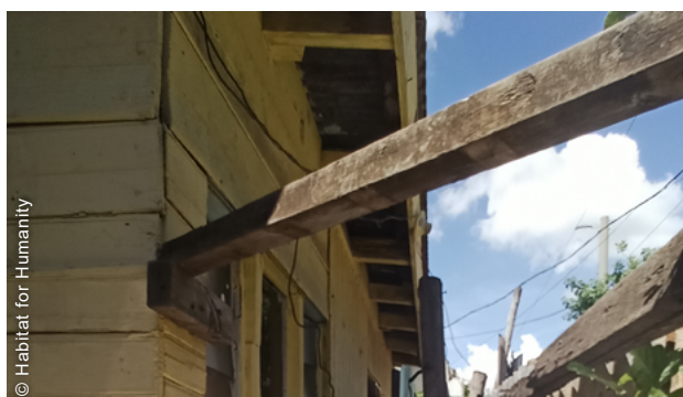
A program review conducted 5 years (and a hurricane) later found that the retrofitted houses were still in good conditions.
