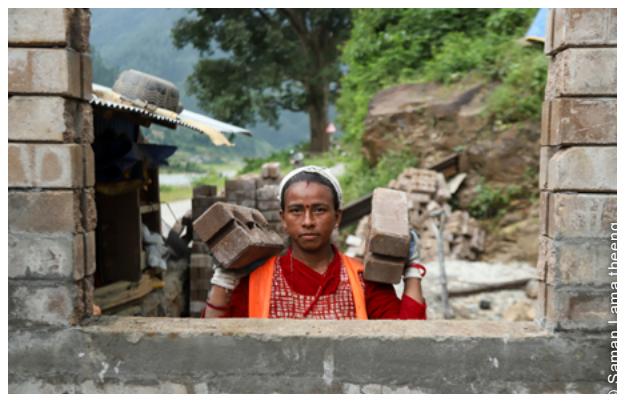
Ms. Babita Rana, a model house beneficiary and worker, transports CSEB blocks, building a safer tomorrow for herself and her community. (Nepal)
