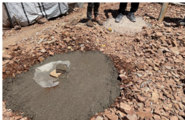
B - Concrete foundation pockets/slabs
