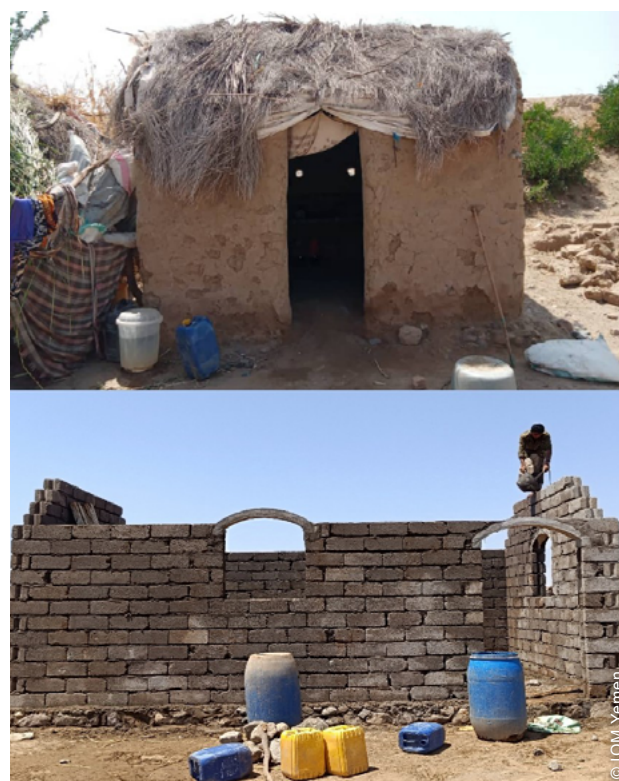
Shelters were upgraded using a cash modality, so that families could implement the works themselves, which built trust with landowners.
