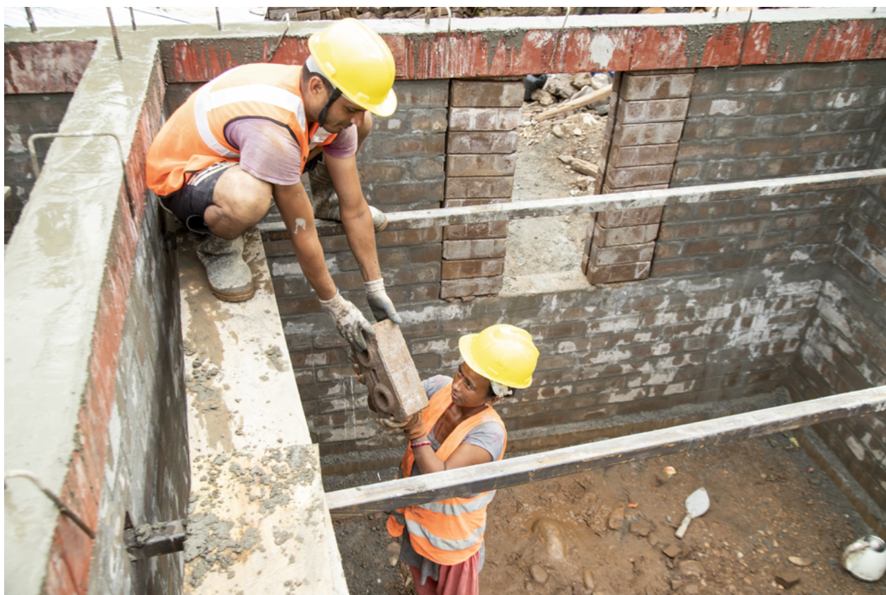
Shelter construction in Nepal.
