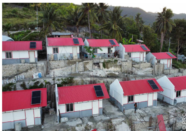
The project targeted households who could not safely return and rebuild on their original plots of land, as they were located on no-build zones.
