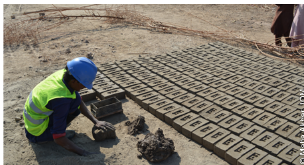
Initially, cement stabilisation in mudbricks was used, accompanied by testing and training. However, it was later abandoned based on household preference.
