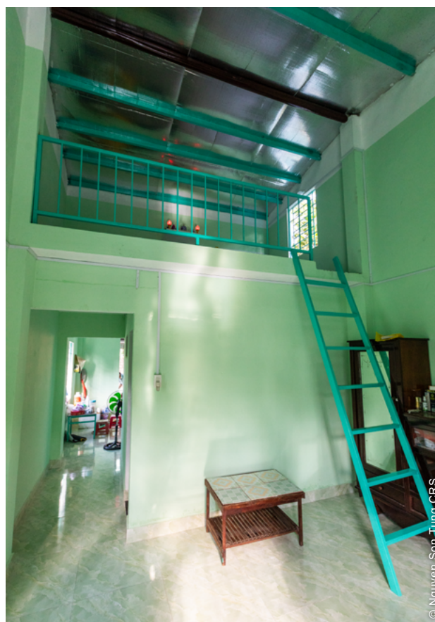
Specific safety measures, such as mezzanines, were incorporated in the project.
