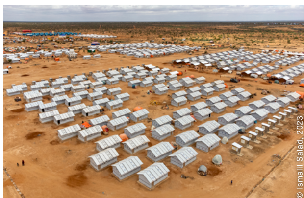
Improved Emergency Shelters (IES) were designed to enable households to incrementally upgrade their shelters over time.
