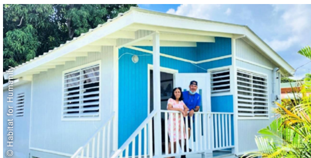
Over 800 houses were repaired, with priority given to walls and roofs, as well as access interventions. Local, safe construction practices were followed.
