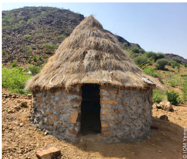
In some locations, families built traditional structures using local materials such as thatch and stone masonry.
