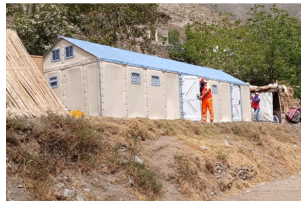
H - Addition of a second door
