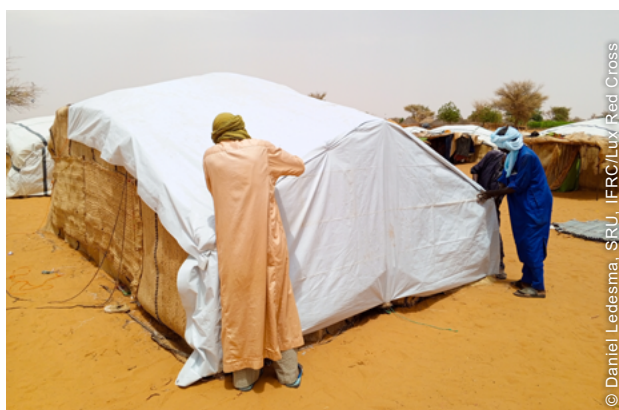
During the field testing phase, following community consultations, the new tarps were distributed and installed in displacement sites in Niger.
