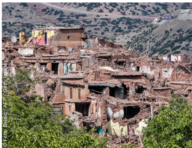
The 2023 earthquake affected many villages located in the High Atlas Mountains near Marrakesh, damaging or destroying approx. 60,000 homes.
