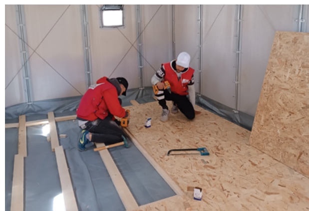
D - Installation of OSB wooden flooring platforms
