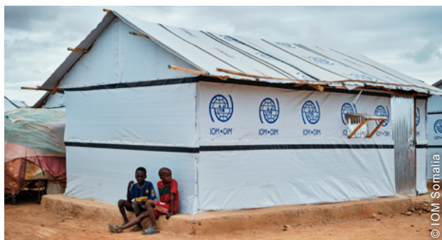
An Improved Emergency Shelter (IES) with raised for an easy upgrade and as a flood mitigation measure.
