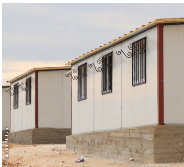
Shelter units were installed over concrete plinths. This typology balanced speed of delivery, thermal performance and durability.
