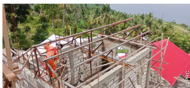
While structural features were fixed, households had a degree of customization on other things, such as the location of the bathrooms.
