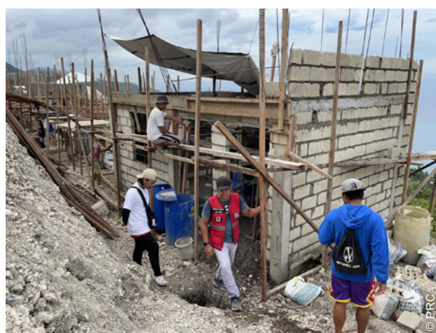
Construction was overseen by project technical staff, local authorities and volunteers.
