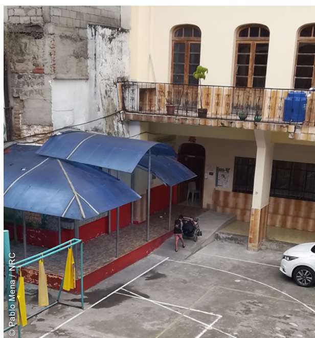
Accessibility features were also implemented, such as ramps.
