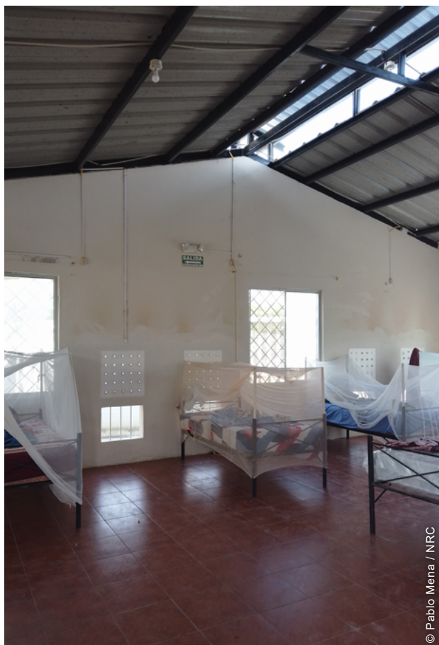
The project selected six communal shelters providing services to migrants, refugees and vulnerable host populations, with the aim to improve habitability.
