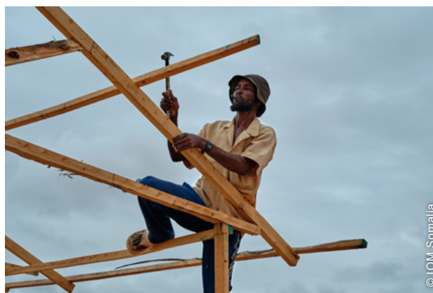
The use of timber frames for shelter construction allowed to erect many units in short timeframes, while also permitting several upgrade options once resources and conditions allowed.
