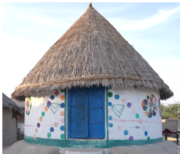
The design choices, including the circular shape and conical roofs, helped reduced the amount of bricks and contributed to budgetary savings.
