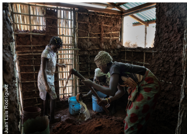
Women taking part in wall-mudding for a shelter construction in Mozambique
