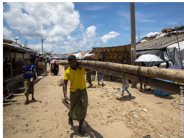
Transportation of bamboo poles for the construction of shelters in Cox's Bazar.
