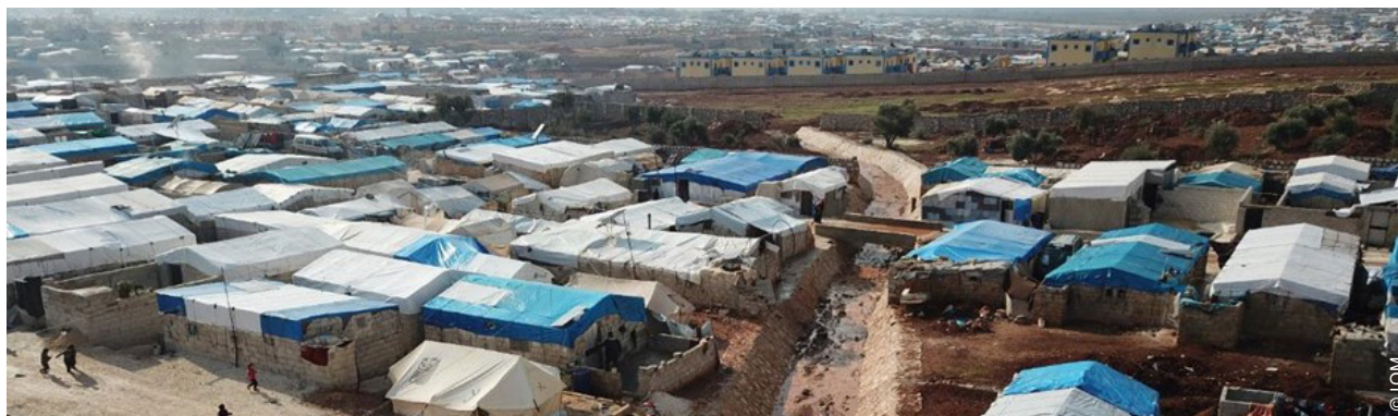
A range of masonry shelters in Northwest Syria.
