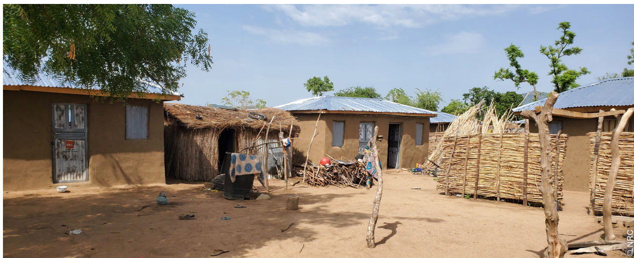
A view of the site with the mud shelters. 340 shelters with two different sizes of 18 m 2 and 21 m 2 were constructed.
