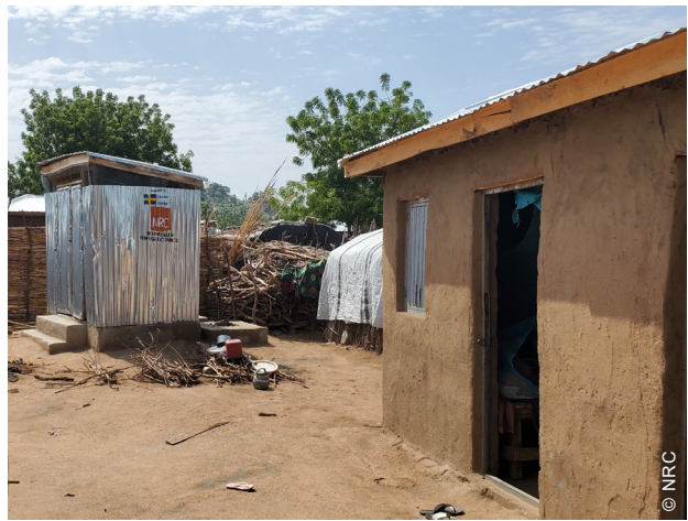
Coordination with the WASH sector for provision of latrine facility.
