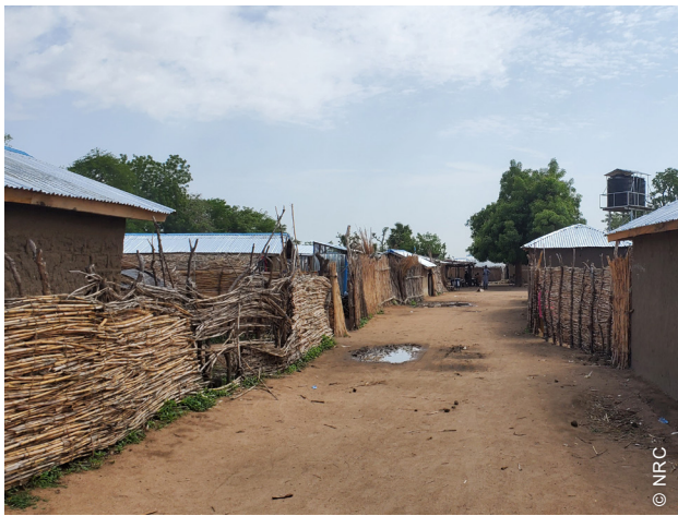
The community was included in the design phase of the mud shelters, ensuring engagement throughout the project cycle.
