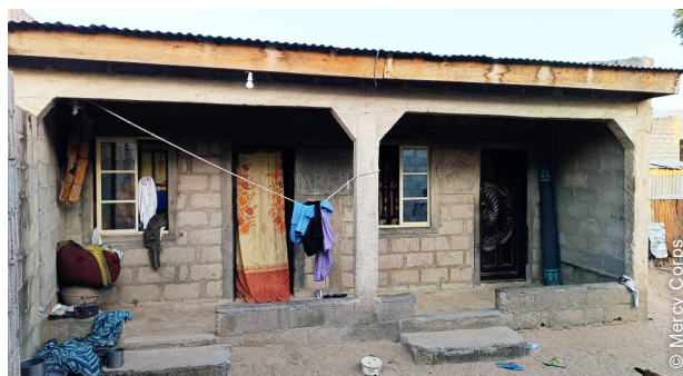
View of a completed shelter with micro solar installation.
