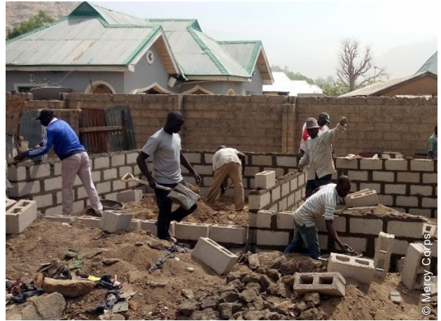
Construction of the permanent shelters using blockwork.
