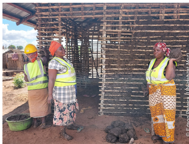
More than 40 women were trained in resilient construction techniques. They were trained in plastering techniques using local mud, December 2021.
