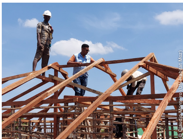
Local carpenters under training on reinforced roof structure connection, November 2021.
