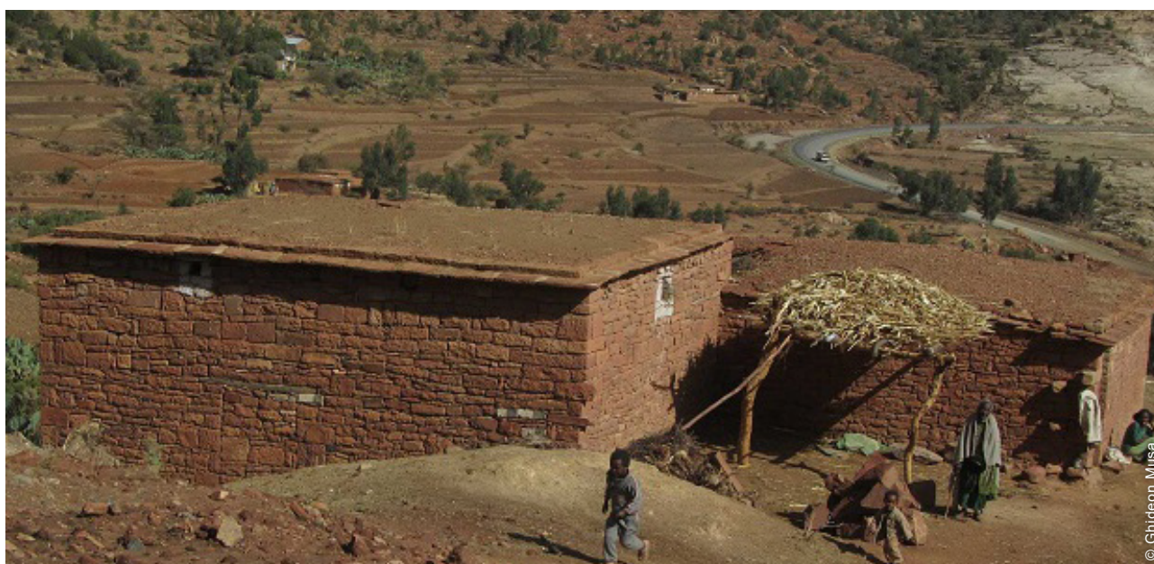
View of a traditional Hidmo house in the Tigray region characterized by masonry walls and flat mud roofs.
