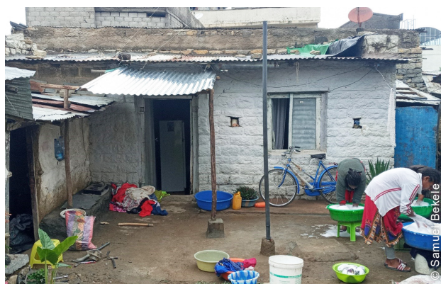
Renovation of roofing and porch in Kedamayweyane sub city, Mekelle.
