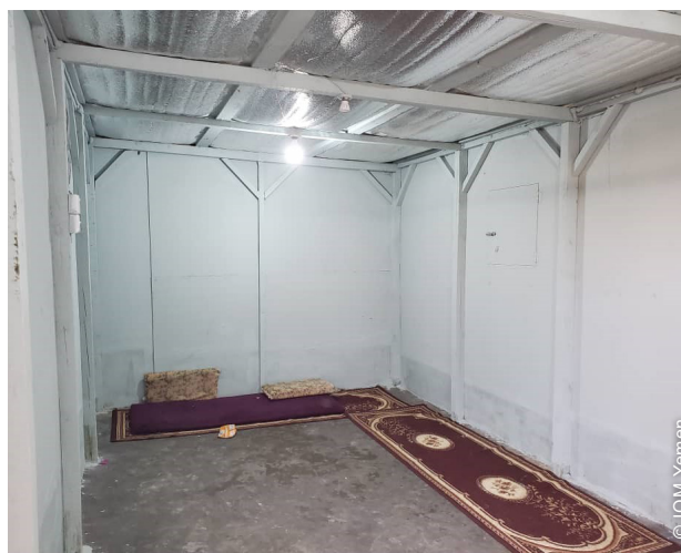
Roof was insulated to protect from the harsh environmental conditions.
