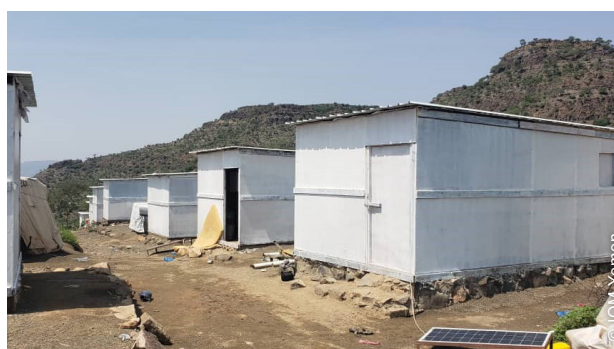
The shelters were painted from the outside for additional protection against water leakage.
