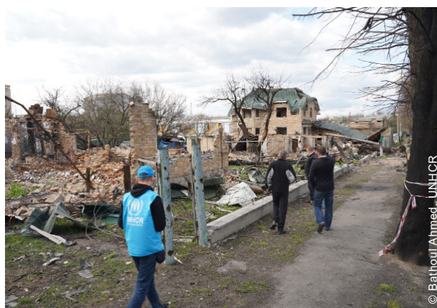
Specialists were consulted and engaged with the Shelter Cluster for debris management prior to reconstruction due to the presence of unexploded ordnance and asbestos.
