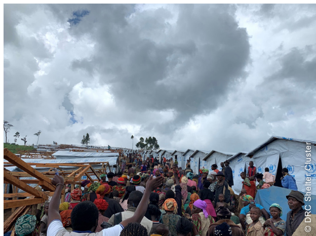
Emergency response - Construction of emergency shelters on site.
