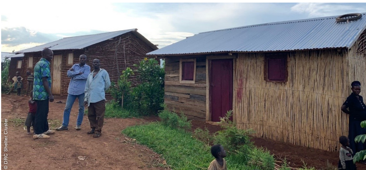
Durable response - Shelters constructed for the returnees using local construction techniques.
