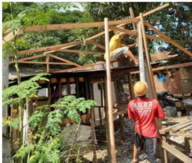
House rebuilding process in October 2022, after Typhoon Rai.
