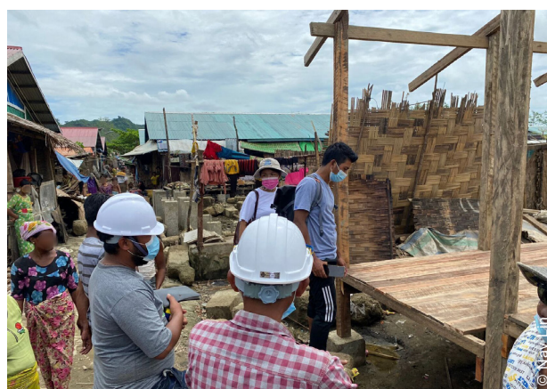
A shelter team inspects ongoing construction works, September 2021.
