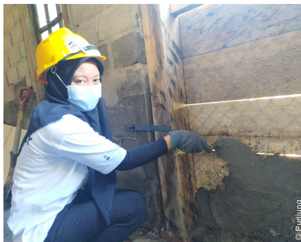
Construction training using retrofitting method (ferrocement) for women in Karampuang Village.
