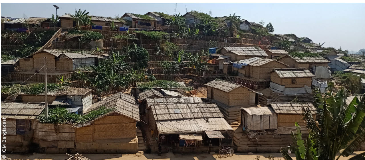
A view of Camp 9 after the reconstruction in April 2022.
