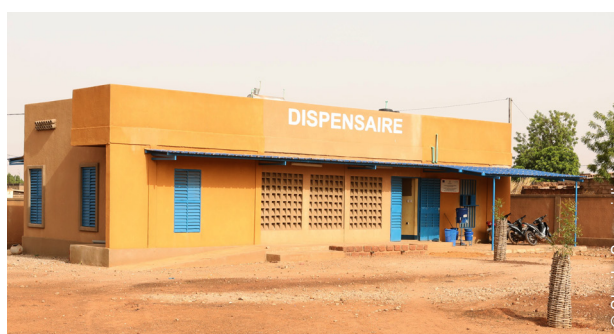
Extension building for Health Center in Dori, March 2022.
