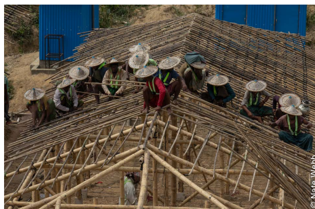
All shelters were constructed by teams of camp residents through Cash-for-Work.
