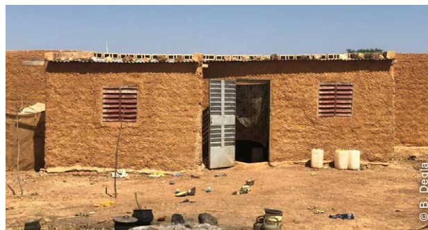
Semi-durable shelter made of mud brick. IDPs are supported with technical guidance and cash for these constructions.
