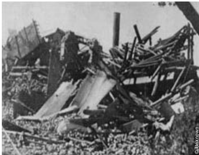
Jinnah road after the earthquake of May 1935. The rubble was completely removed in December 1936.
