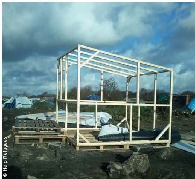
The organization started using a shelter design at the end of September 2015. Frames were prefabricated off site and, for the most vulnerables, shelters were set up by volunteers.
