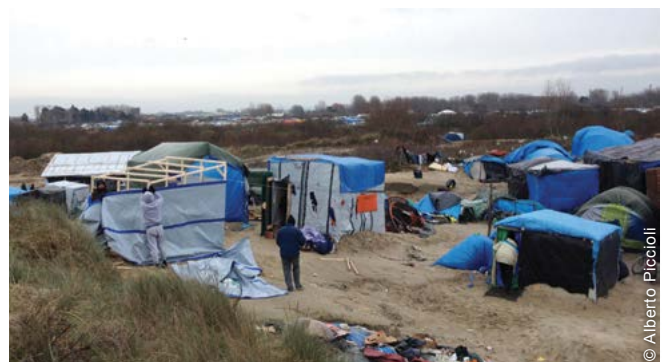
The organization started using a shelter design at the end of September 2015. Frames were prefabricated off site and built by volunteers only for the most vulnerable.
