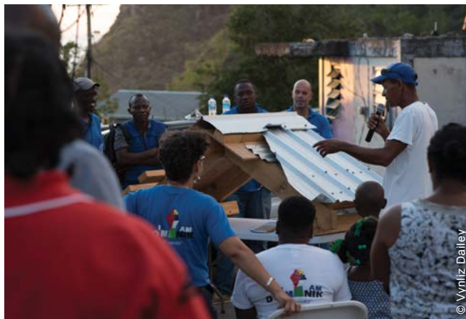
A model was used to explain safe roof repair interventions.
