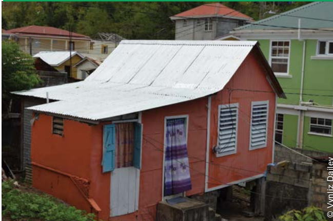
Forty migrant labourers were employed to work on the project thanks to a partnership with another organization that supported their recruitment and training.
