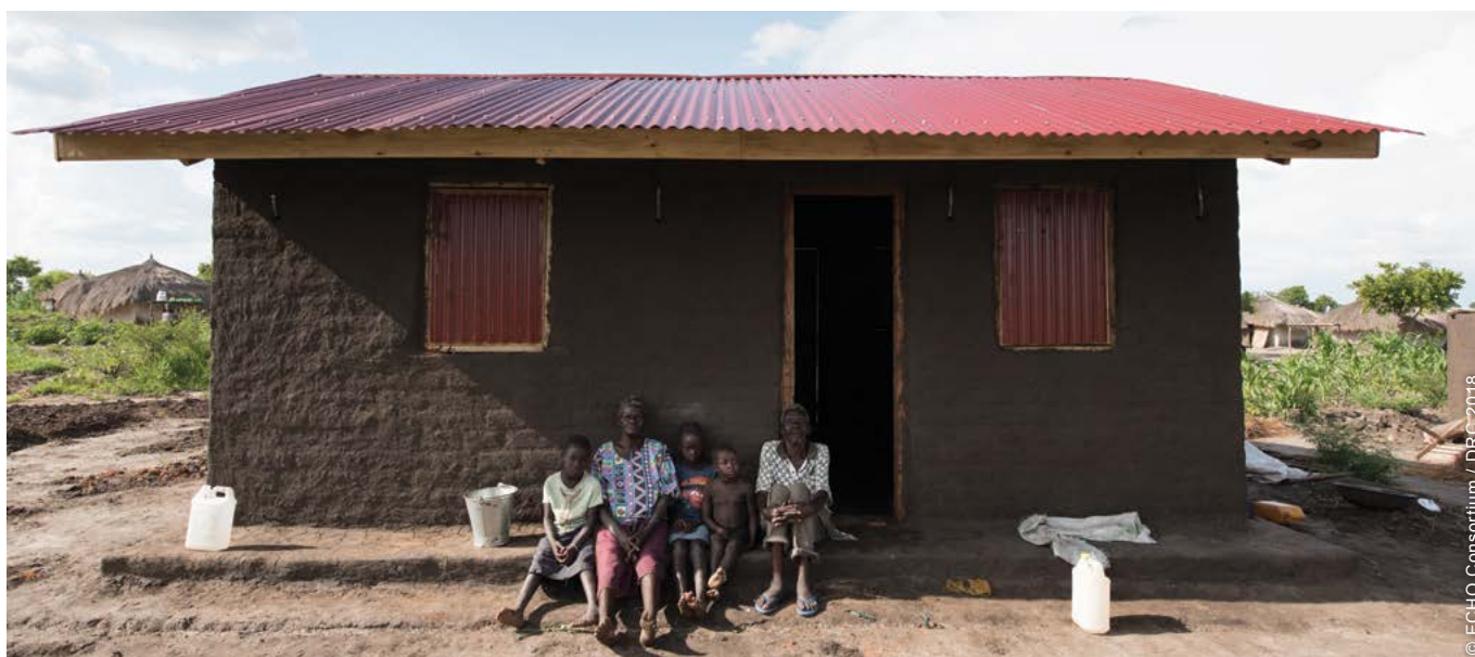
Shelters were built with locally available materials through the engagement of local youth groups who were divided in different teams based on their skills.
