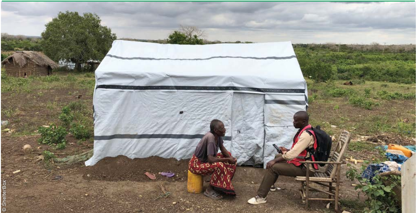
Survey findings informed subsequent distributions. While personal safety and protection from the rain were largely met, shelters performed poorly against the heat and the cold temperatures. Some items, such as mosquito nets, were seldom used as was expected.
