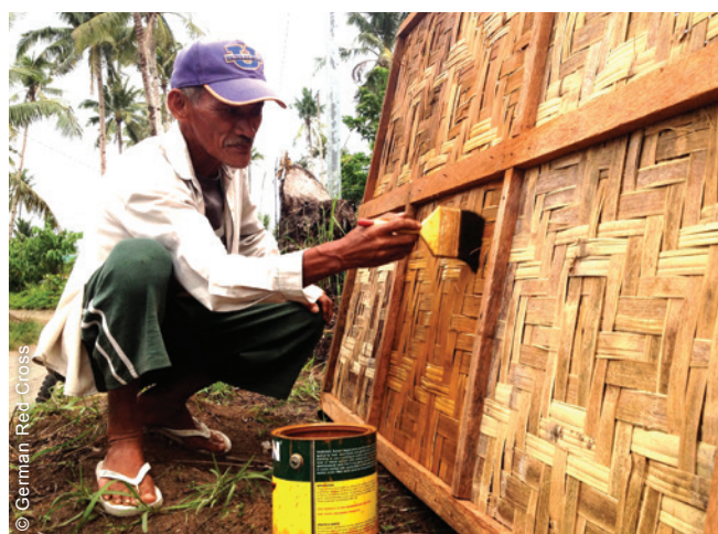
In some projects, materials were treated to improve the durability of the shelters.
