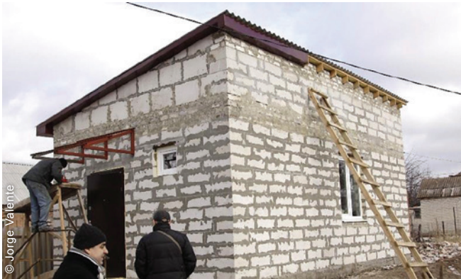
Some projects aimed at re-building completely destroyed houses (Sloviansk).
