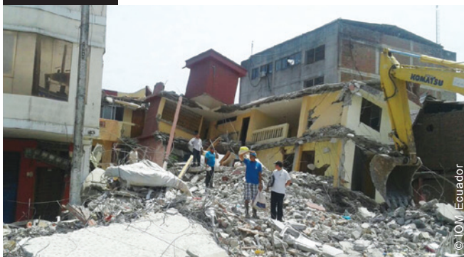
The urban area of Portoviejo was particularly affected by the earthquake. Here is an image of the centre, soon after the first earthquake in April 2016.
