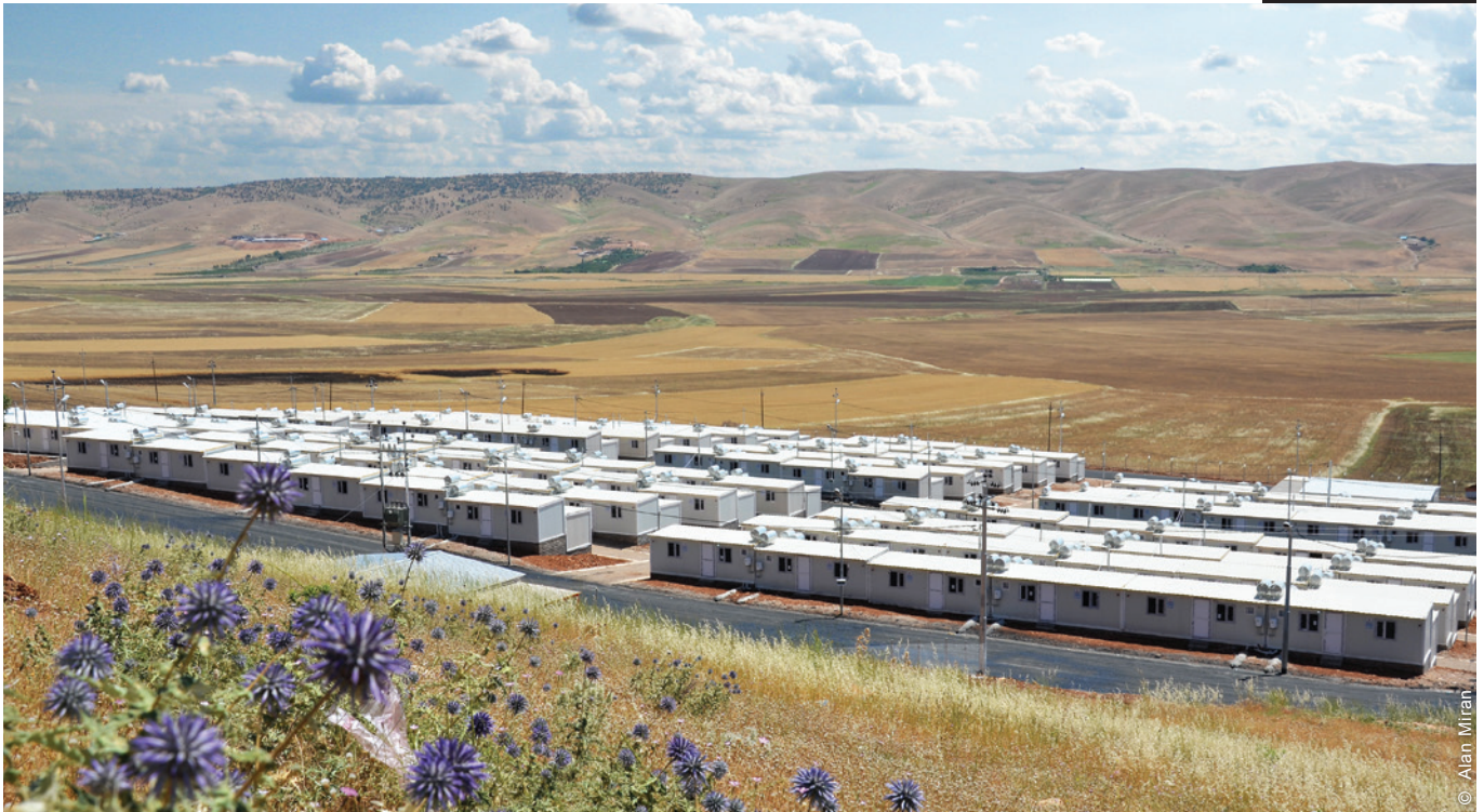
The project planned and built four sites equipped with durable, prefabricated, shelter units for vulnerable IDPs across the country (here, the Darkar Ajam site).
