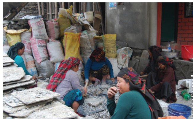
After the rapid gender analysis, the project consulted the communities, engaged women in construction activities, and aimed to meet specific gender needs in both distributions and construction (here, on a building site in Barpak).
