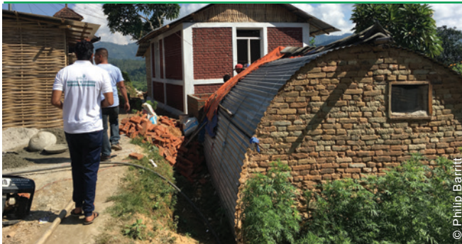
Temporary shelters, built with the materials provided, bridged the gap during reconstruction of more permanent houses (here, in Kavrepalanchok district).
