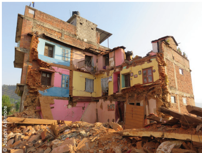
The earthquakes caused massive destruction of public buildings and housing.
