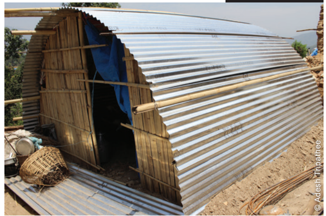
Some people used the materials provided to build temporary shelters according to the organization's design.
