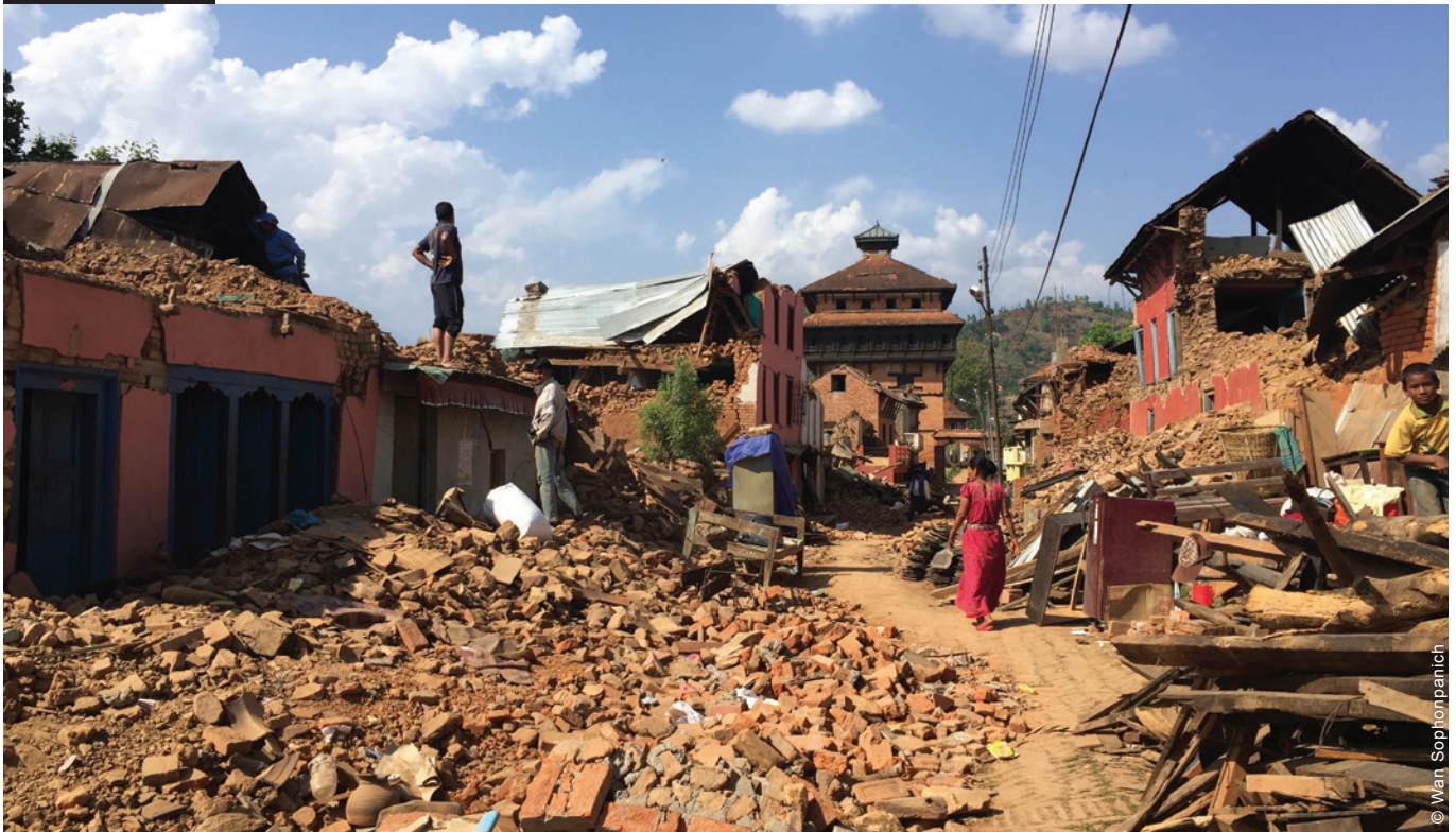
The first step in the response is to assess the damage, and then clear the rubble to allow recovery efforts to start.
