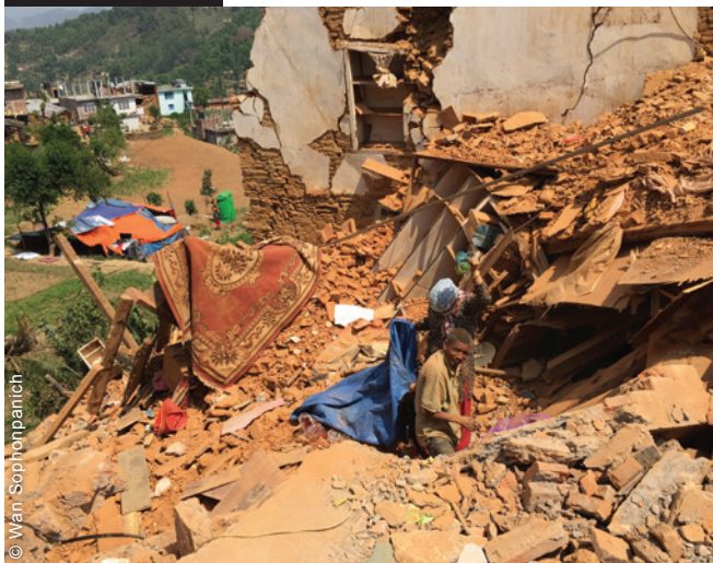
People salvaged personal belongings from destroyed houses.
