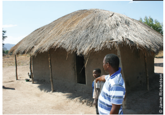
Many of the traditional houses withstood the floods, as they were built with contextually appropriate features, such as roof overhangs and raised platforms.
