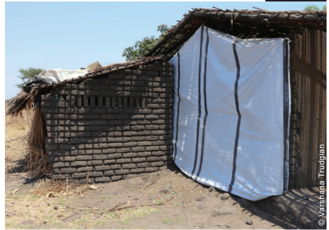
Tarpaulins from the shelter kits were used, amongst other purposes, to seal off damaged parts of the houses.
