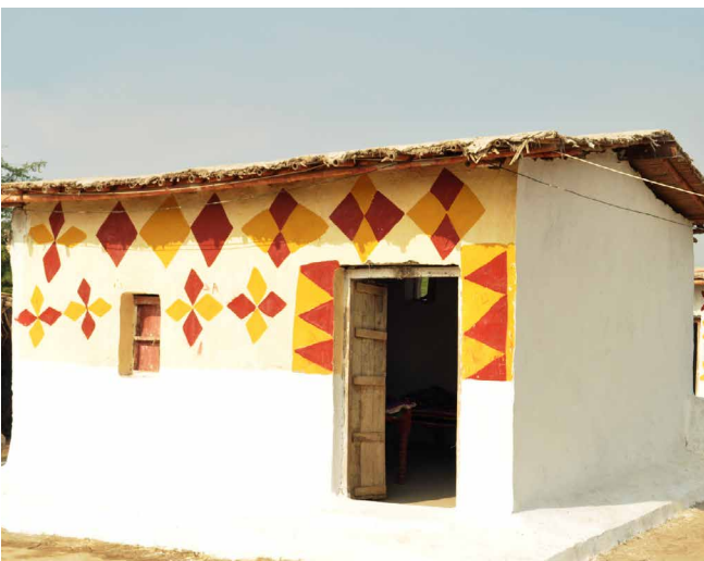
Sangar district, Southern Sindh, December 2013. Lime stabilised mud brick foundations and walls. Flood resistant with pitched, not flat, roof. Photo: Magnus Wolfe Murray
