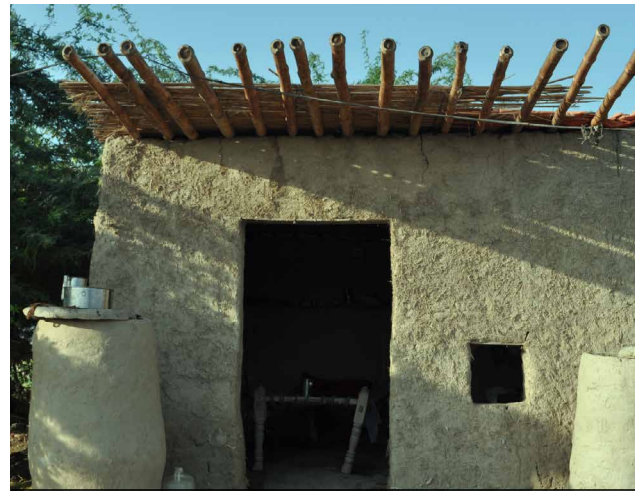
The second, transitional stage in the life of a roofing kit. This temporary hut, lived in for about a year, will be dismantled and the roof will be used for a permanent house. This saves around US$ 111 from the cost of the new shelter. Photo: Magnus Wolfe Murray
