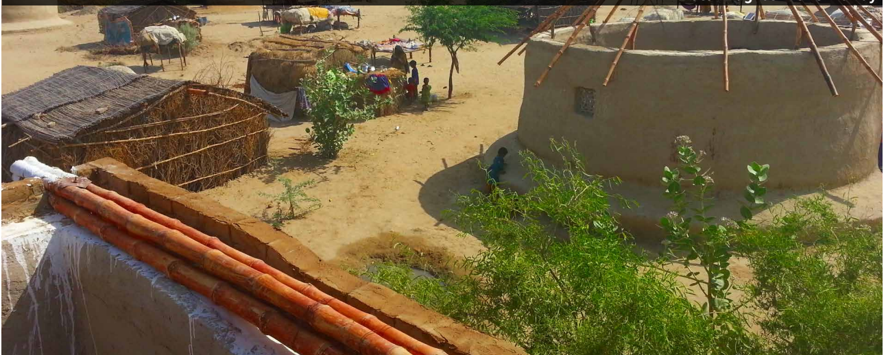
Two different types of shelter: in the foreground, an unfinished, square, flat-roof house with compound bamboo ring beam on top of the walls. To the right, a round house (known locally known as "chulla"). This was the first time people in this village had constructed permanent shelters. Photo: Magnus Wolfe Murray
