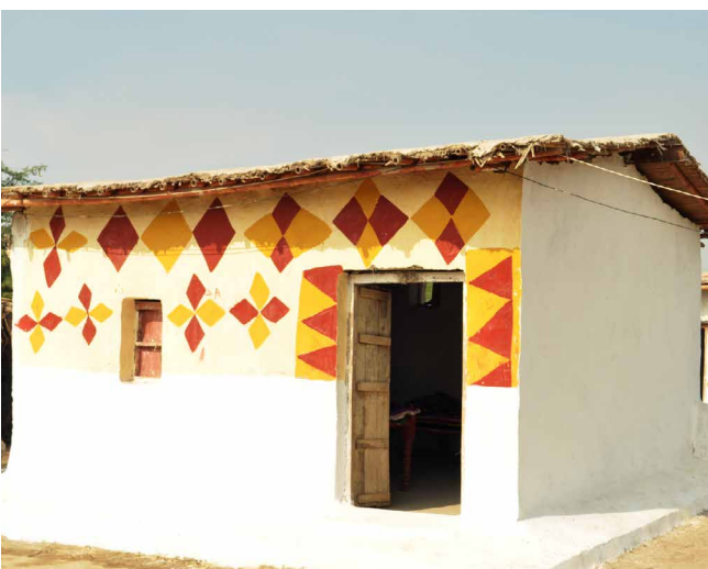
Sangar district, Southern Sindh, December 2013. Lime stabilised mud brick foundations and walls. Flood resistant with pitched, not flat, roof. Photo: Magnus Wolfe Murray
