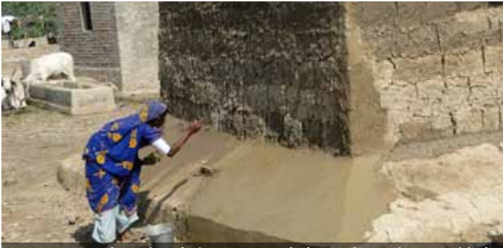
Women plastering their one room shelters. The project provided cash to build shelters and training on safer construction with incremental improvements such as stronger plinths and footings to walls. Households chose their own shelter design.
