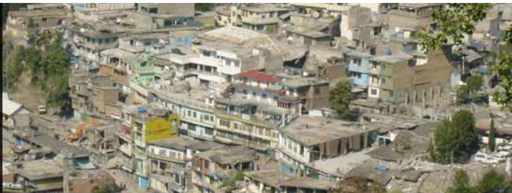
Muzafarabad, Pakistan 2005 after an earthquake. Photo: Joseph Ashmore
