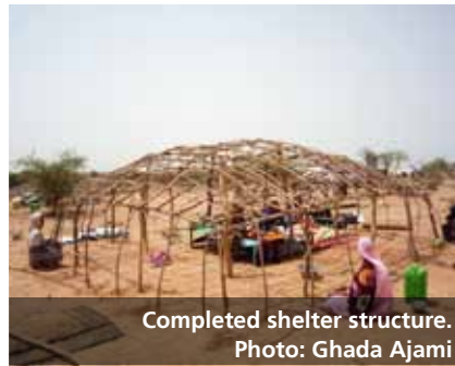
Shelter structure under construction. Photo: Christian Jepsen
