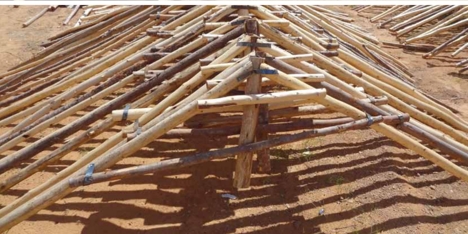
Top: View of a camp before construction. Each organisation established a large workshop in each camp to store materials and prefabricate components. Images: Joseph Ashmore
