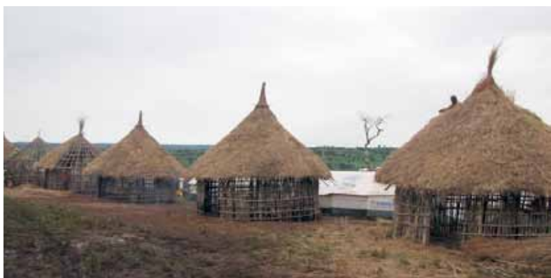
Timber and bamboo frames shelters were built with thatched roofs as a more durable shelter solution than tents. It proved challenging to source mud to plaster the walls as originally intended. Photos: Left: UNHCR, Right: Demissew Bizuwerk / IOM Ethiopia.
