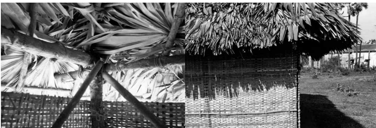
Details of a model home built out of bamboo and thatch to explain a safer techniques in cyclone resistant housing. It had key elements of: a well-anchored central post, triangulation to stiffen the frame, good connections of roof to wall using metal connections Photos: Ian Davis
