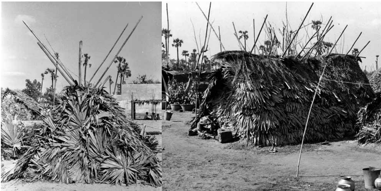
The government made stocks of thatch and bamboo available so that families to improvise shelters. Non-governmental organisations also built many thousands of these shelters. Photos: Ian Davis
