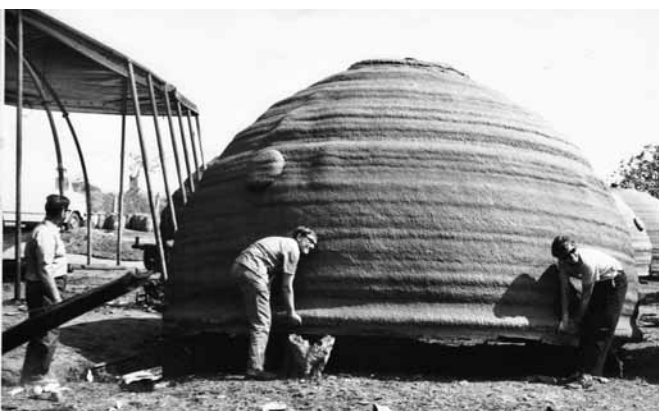
Above and Centre: polyurethane igloos arrived too late to satisfy emergency shelter needs. Similar shelters were also deployed in Turkey (Gedez, 1970 and Lice 1975) and Peru (1970). they were finally abandoned as a system following the experiences in Lice (1975) Photo: Ian Davis
