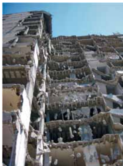
Where buildings had many tenants - different apartments were assessed separately from the building Photo credits: CHF
