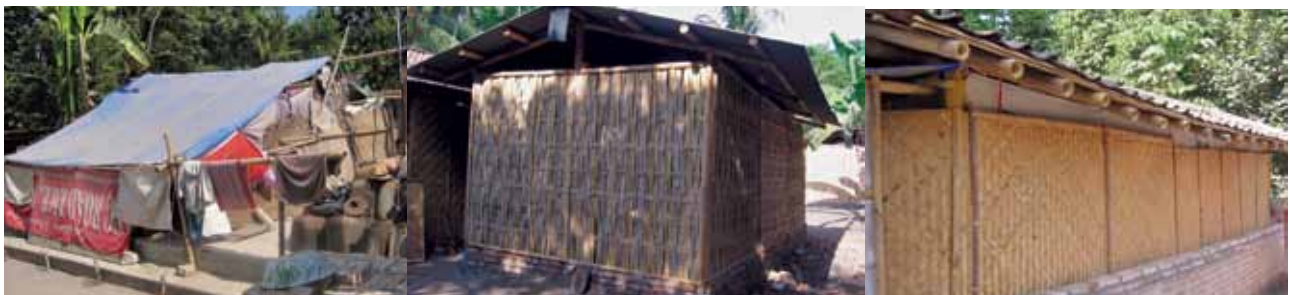
Left: plastic sheeting was distributed during the emergency phase. Centre and right: small grants were provided to help build transitional shelters. Many different and innovative designs were built. Photo Dave Hodgkin
