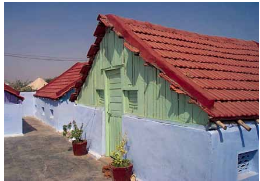
These school buildings were adapted from the transitional shelters. The low walls reduced the risk of masonry falling on occupants during future earthquakes. Photo: Chris Cattaway
