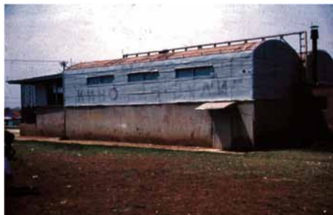
US army Quonset huts built after the earthquake. Top image: taken in 1974, 11 years after the earthquake. Bottom image: taken in 1987, 25 years after the earthquake. Two of these huts had been elevated and joined together to form a small cinema.
