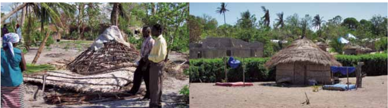
Left: a damaged house. Right: self-built reconstructed house using items distributed. Photo: Lizzie Babister
