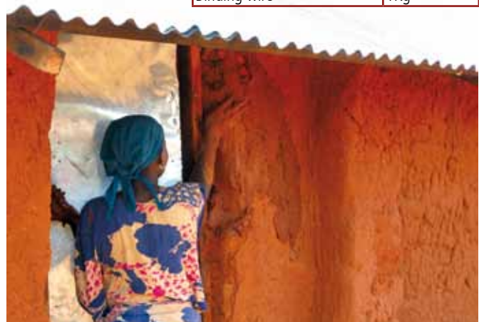
Shelters under construction in Dadaab. Much of the construction, including making mud blocks, is done by the women. Photo: Jake Zarins
