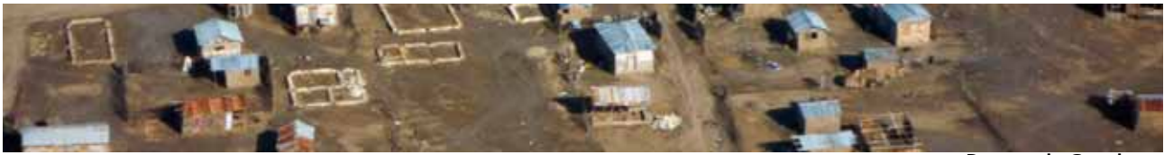
Damage in Gonaïves Photo: Joseph Ashmore
