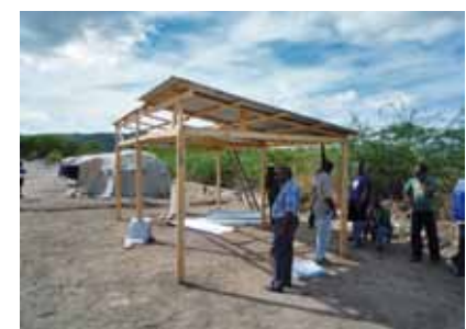
Prototype transitional shelter Photo: Joseph Ashmore
