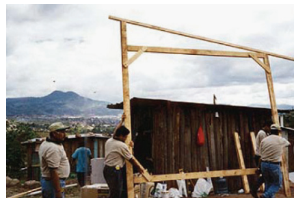
Shelter assembly using prefabricated walls
