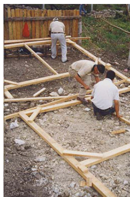
Prefabricating walls
