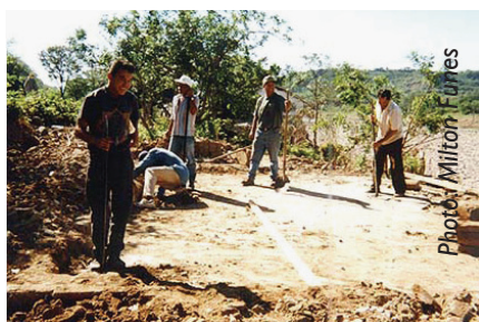
Marking out the site for a shelter
