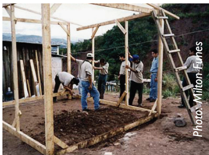
Completing the frame
