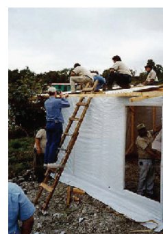
Covering the roof with corrugated iron
