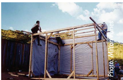
Covering the frame
