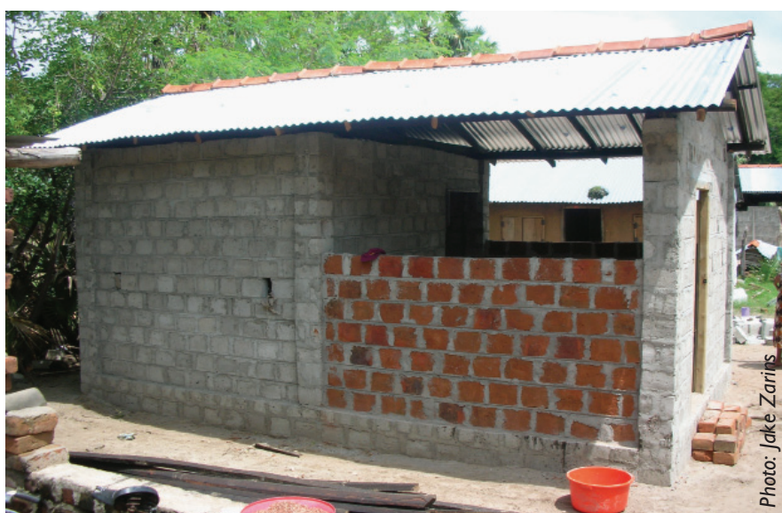
A durable upgrade of a core shelter
