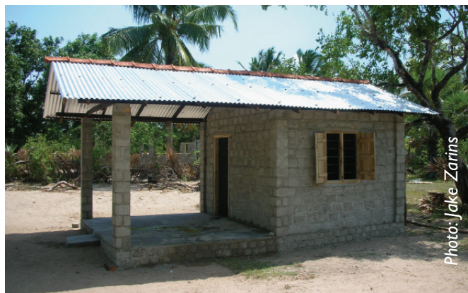
Completed core shelter
