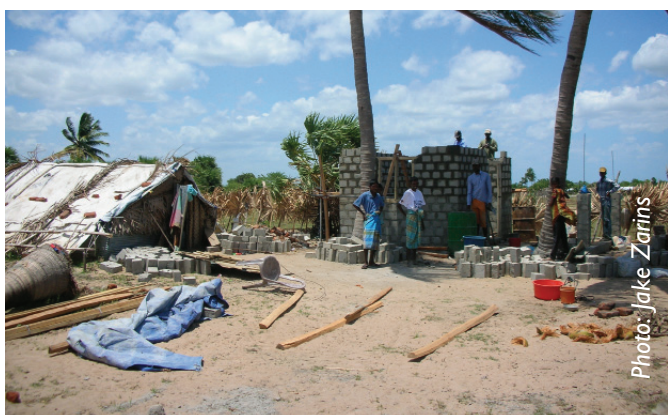
Core shelter under construction
