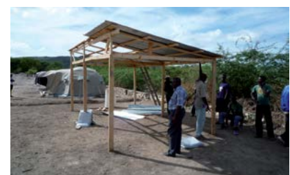
Prototype transitional shelter Photo: Joseph Ashmore
