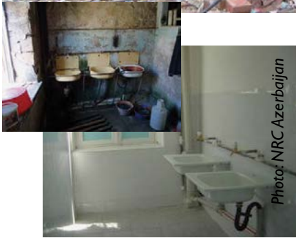
Bathrooms before and after upgrade
