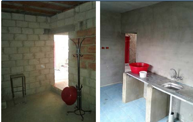
Where required, works included rehabilitation of household-level water and sanitation systems.
