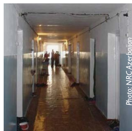
Corridors before and after upgrade
