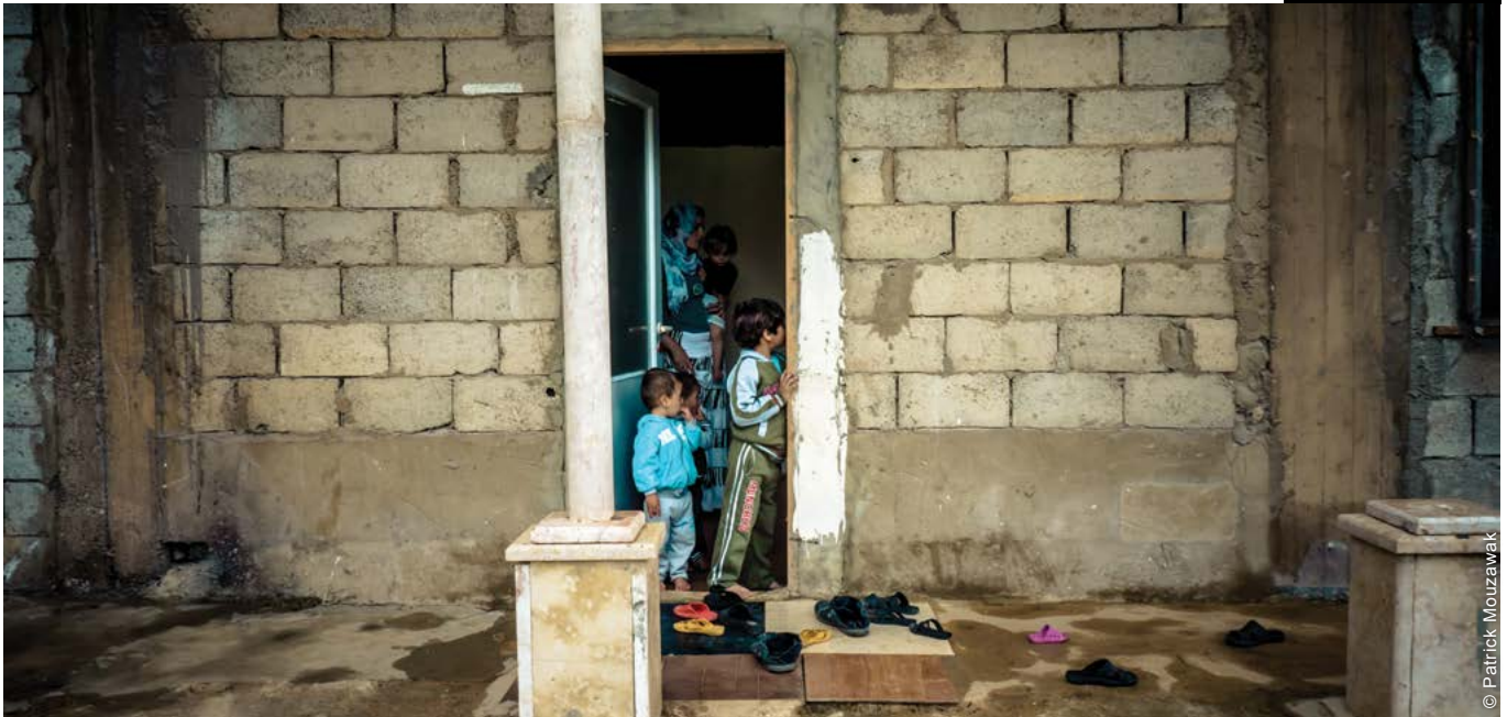
The majority of refugees in Lebanon stayed in rented accommodation. High housing demand, combined with the high cost of living, led to many people living in substandard and overcrowded conditions.
