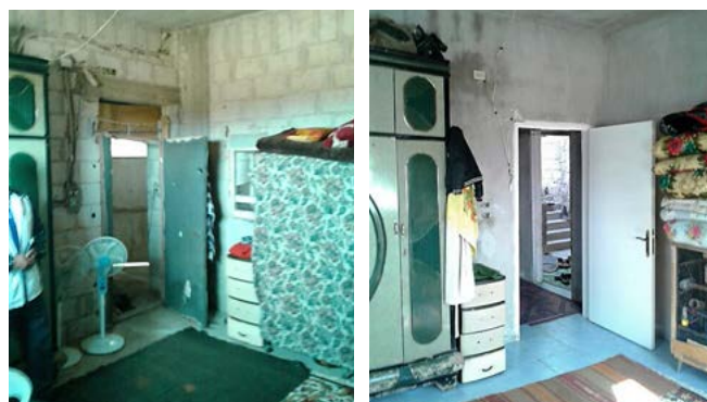
Rehabilitation works were conducted using local labour and materials.
