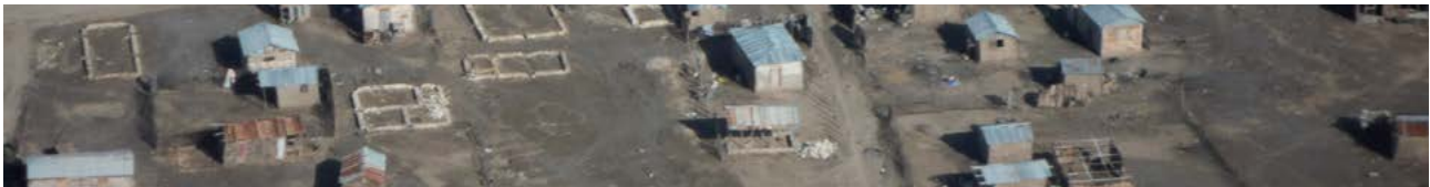
Damage in Gonaïves Photo: Joseph Ashmore
