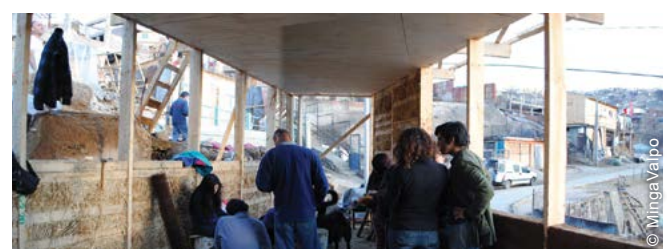
Local groups of architects organized building workshops to rebuild some of the houses affected by the fire on the Quebradas.
