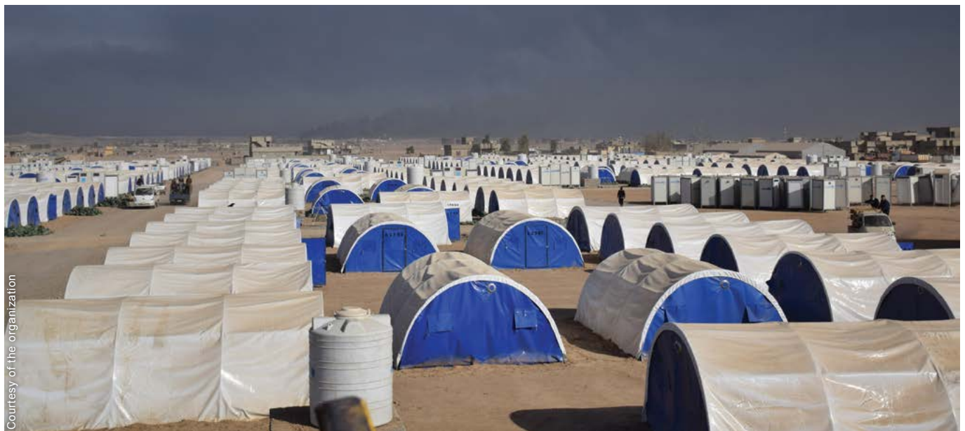
Government standard tents of 6x4m were installed in clustered blocks of 20 each. Space for extensions was minimal but, after families had moved in, upgrades were conducted to the floor and electricity was installed. Partners could then build service facilities in specific blocks pre-allocated in the site plan.
