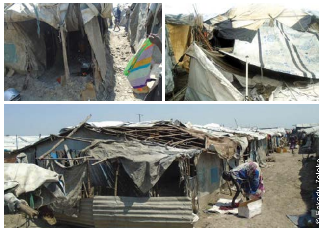
Before rehabilitation, the site offered very poor shelter conditions and was overcrowded, with related fire and safety risks for its residents.
