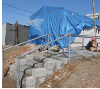
Works also included mobility upgrades within plots or across the camps. From left to right: Concrete pathway and railing leading from shelter to shared/communal latrine. Concrete slab improving wheelchair access. Handrails, concrete stairway and pathway around or between shelter plots.
