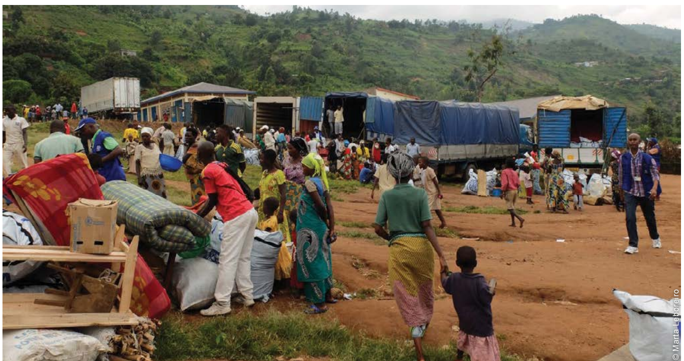
To facilitate the decommissioning process, the organization provided transport assistance and a cash-for-work grant for the dismantling and cleaning of tents and family plots in the camps.
