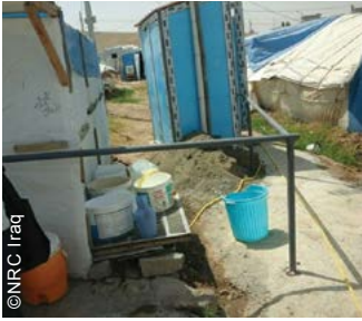
Works also included mobility upgrades within plots or across the camps. From left to right: Concrete pathway and railing leading from shelter to shared/communal latrine. Concrete slab improving wheelchair access. Handrails, concrete stairway and pathway around or between shelter plots.
