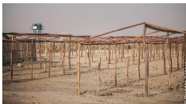
Shelter frames were built by contractors.
