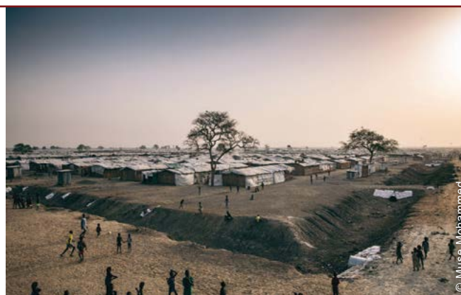
The site works were based on a Dutch “polder” system. They included 28m 2 section drainage ditches, berms, water retention basins, and large volume pumps to evacuate water.
