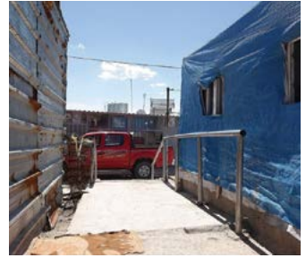
Works also included mobility upgrades within plots or across the camps. From left to right: Concrete pathway and railing leading from shelter to shared/communal latrine. Concrete slab improving wheelchair access. Handrails, concrete stairway and pathway around or between shelter plots.
