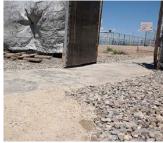
Works also included mobility upgrades within plots or across the camps. From left to right: Concrete pathway and railing leading from shelter to shared/communal latrine. Concrete slab improving wheelchair access. Handrails, concrete stairway and pathway around or between shelter plots.
