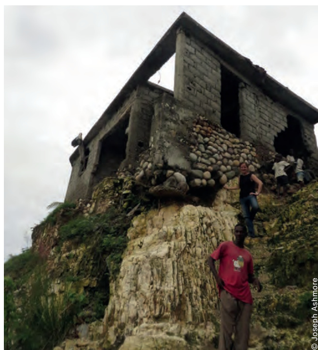
Houses in informal settlements are often vulnerable due to poor locations (marginal sites), poor materials (here we have river stones for foundations) and poor construction.
