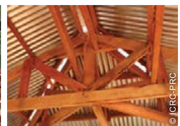
The project used locally available materials (e.g. the amakan sheet, left) and safe construction techniques, including bracing, strong trusses and roof strapping.
