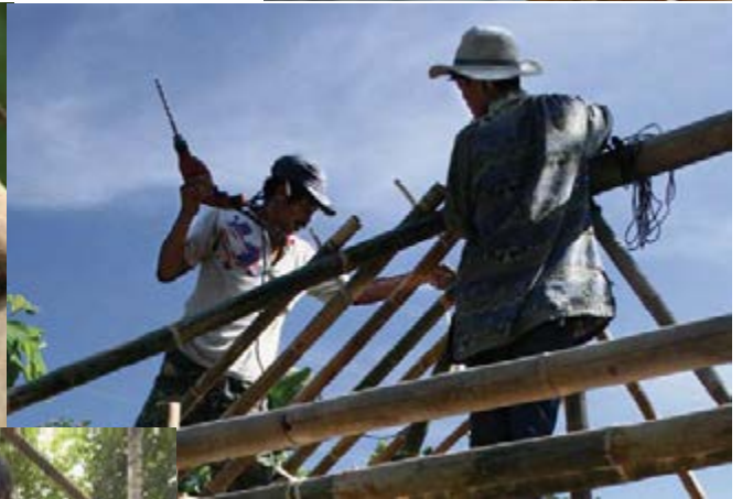
Electric power drills used to drill holes in the bamboo so that it can be pegged
