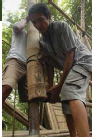
Connecting a vertical post to the foundation
