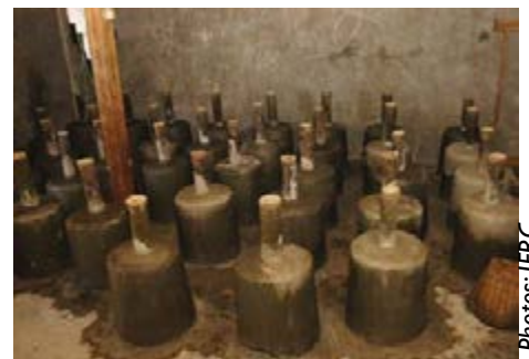
Foundation pads cast with bamboo to connect them to the frame
