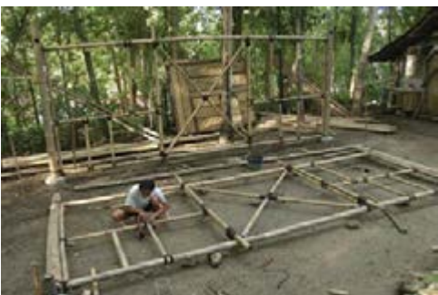
Prefabrication of a wall panel
