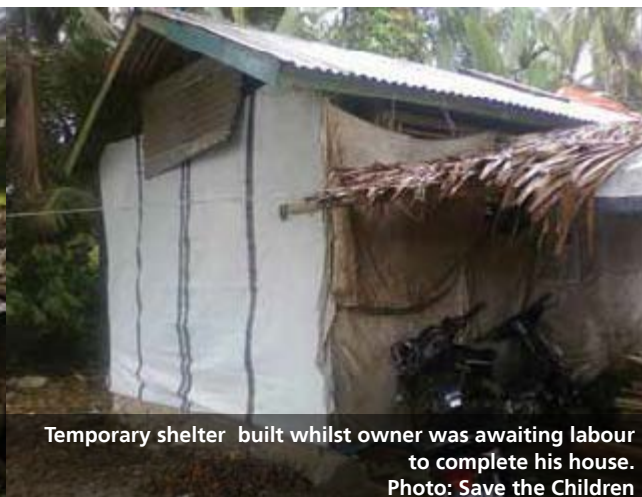
Many materials could be salvaged. Cash grants allowed people to pay for materials and labour according to their needs.
