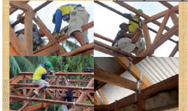
The project had a strong focus on safer construction techniques.
