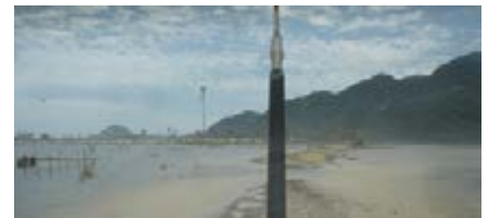
Road shown two years after the tsunami. Access was initially difficult along much of the west coast of Aceh.
