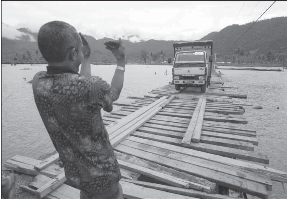
The bridge near Lamno, in Aceh Province, Indonesia, has survived for over a year now, hand built by villagers from coconut palms felled in the tsunami.
