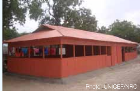
Somalia: storage space in between classroom as acoustic separation
