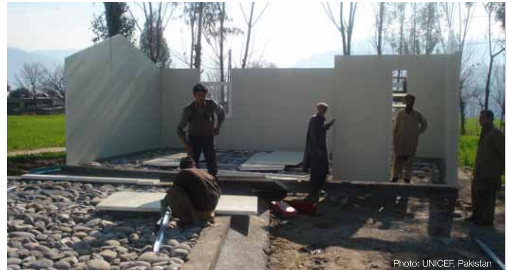
Assembly process of prefabricated wall elements
