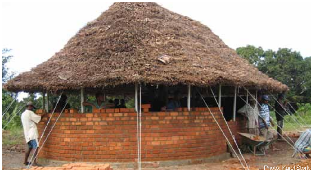
Updating with external brick wall around the tent structure
