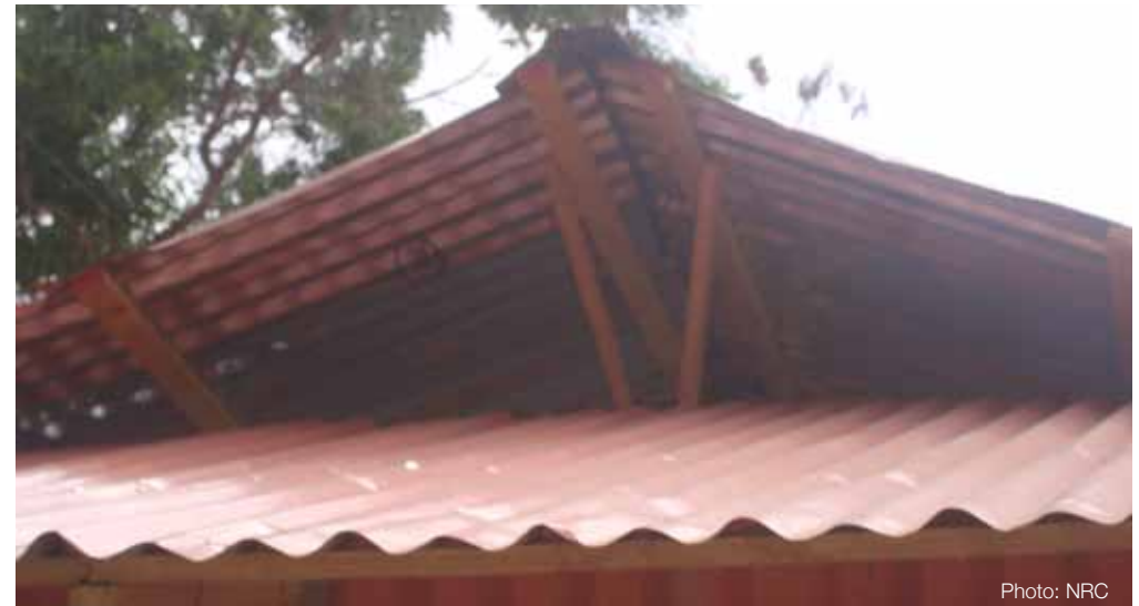
Roof ventilation detail
