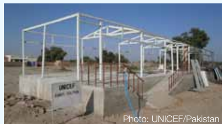
Photo: UNICEF/Pakistan Pakistan: raised floor level to prevent flooding
