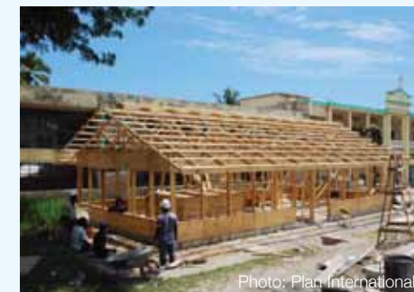
Haiti: Crew of young Haitian construct TLS
