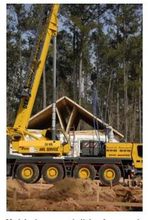
Modular houses are built in a factory and transported to a lot. A crane places the modular on its permanent foundation.
