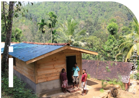
Local environmental damage is long-lasting
